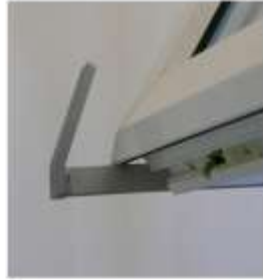
Sash not raising sufficiently to sit on the Sashmate Bracing Arms.
