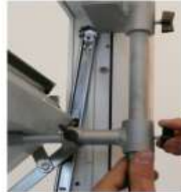
Undo the thumb screw to the Pin and Sleeve. Drop the Pin and Sleeve down 20-30mm and re-tighten thumb screws. Do the same on the second tool.
